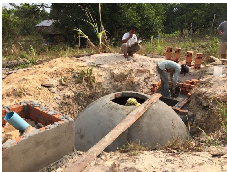
Figure 4.2 Bio-digester building in Toul Korki, facebook: Vanny Lou, April, 2016.
